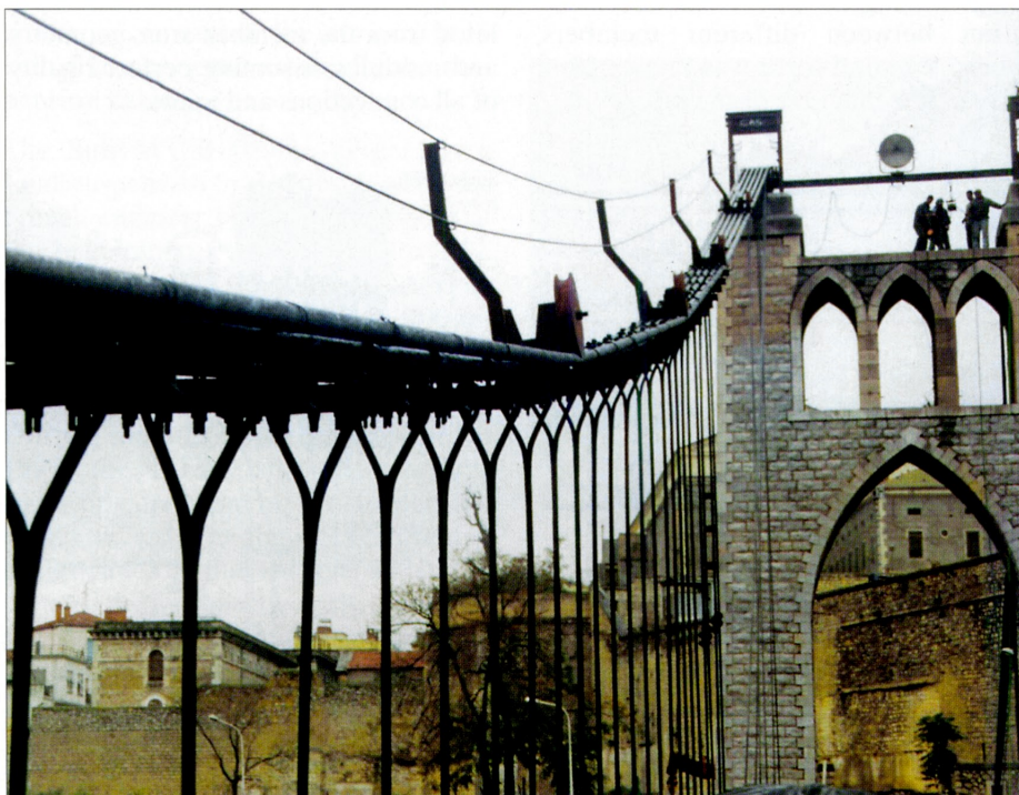
Fig. 6: Pulley and catwalk system along the main cables
