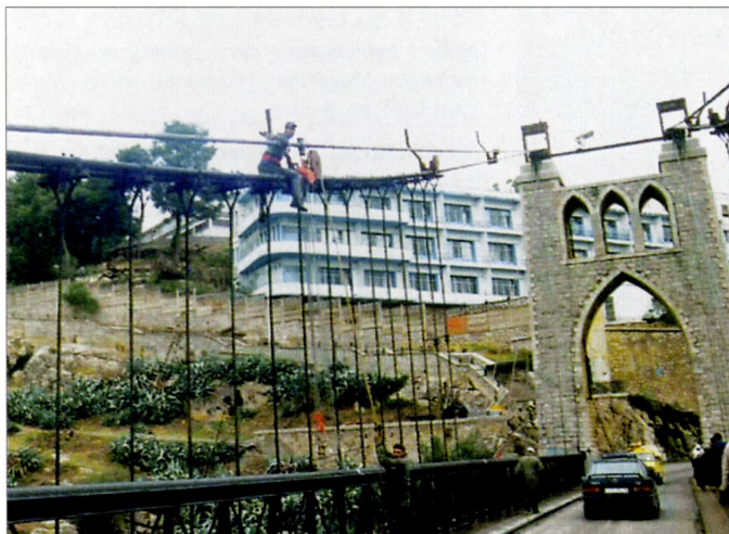
Fig. 8: Releasing the rope from under the pulley
