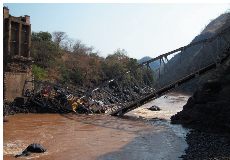
● Fig. 2 - La trave reticolare recentemente crollata. ● Fig. 2 - The trestlework beam that recently collapsed.
