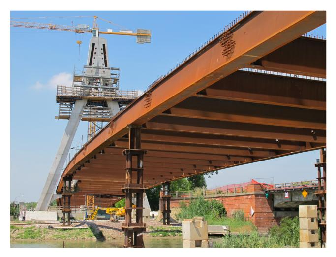
Fig. 5: The steel deck
