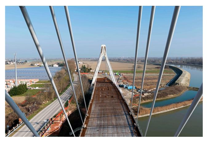
Fig. 7: The deck slab under construction
